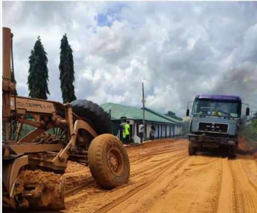
Construction of Ekpena Road has commenced.
